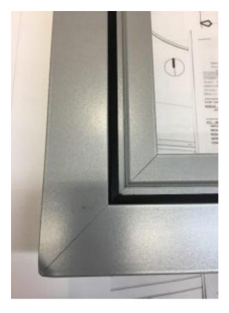
TYPICAL MECHANICALLY FASTENED SYSTEM WITH VISIBLE ATTACHMENT SEAMS & CUT LINES.
